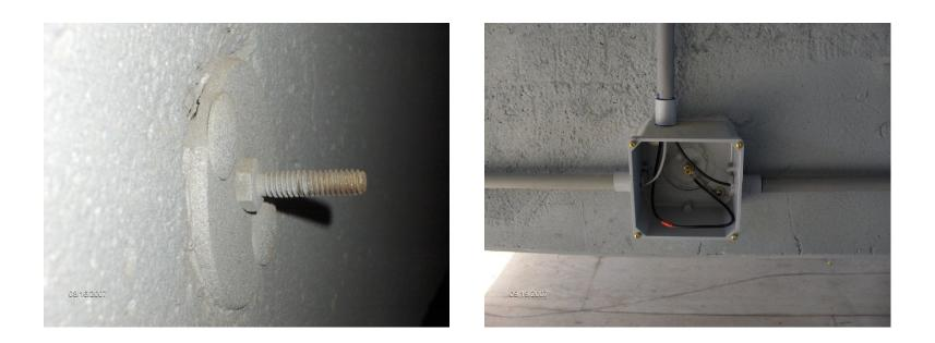
Includes installation of anode terminal plates.
