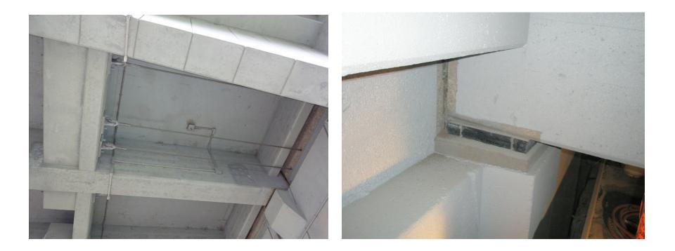
Since the 1990s ODOT has been installing Phase 1 seismic retrofits (keep superstructure seated on substructure) on historic coastal bridges. The bearing seats are extended, rocker-type bearings are replaced with elastomeric pads, lateral shear blocks are added, and longitudinal cables tie the spans together.
