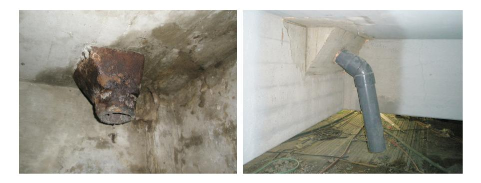
Existing small-diameter drains are replaced with 203 millimeter (8 inch) diameter PVC drains with modern inlets.
