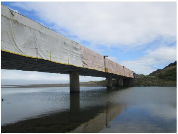
Includes work platforms and containment. Safespan work platform is shown with containment provided by tarps.
