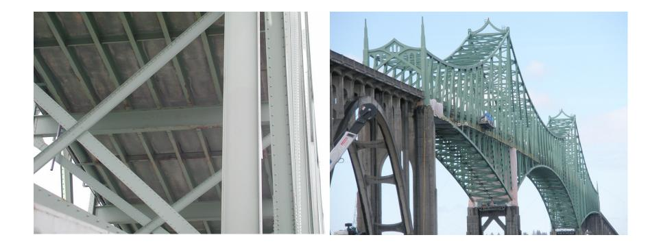
The bridge recoating project was completed in 2001 with less than satisfactory results. The bonding company paid on warranty and ODOT applied the funds to coating repairs performed during South end cathodic protection project.
