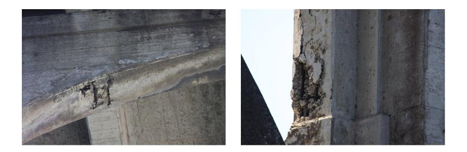
Marine salt damages the reinforced concrete by providing electrolyte and a catalyzing effect for corrosion of reinforcement which in turn causes spalling of concrete.
