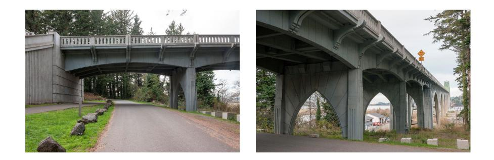
The south approaches of the bridge received impressed current cathodic protection between 2007 and 2012. This project included coating repairs resulting from 2001 project, cathodic protection, Phase 1 seismic retrofit, larger bridge drains, "stealth" rail, expansion joint seal replacement, and sealing/overlay of wearing surface. Construction cost \$30.0 Million.
