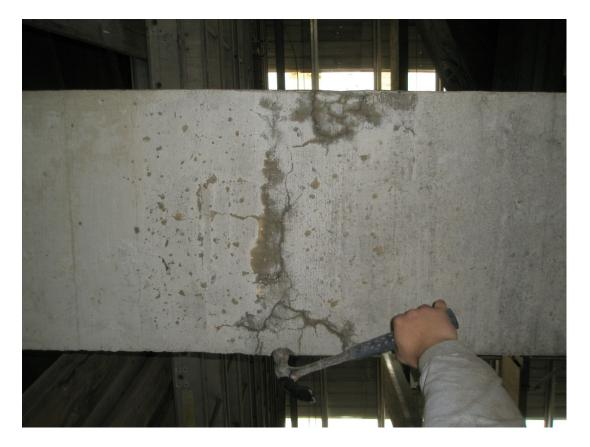
Includes visual inspection and sounding of concrete to identify spalled or delaminated areas.
