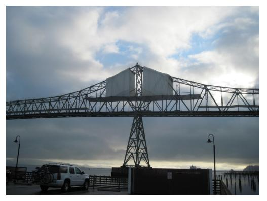
Structural steel repaint cycle is about 15-20 years in the marine environment, less with poor workmanship. ODOT prefers abrasive blast surface preparation to SSPC SP-10, and recoating with 3-coat moisture-cured urethane system with zinc in the primer. Corroded rivets are replaced with high strength steel bolts, and sometimes there is a need for repair of section loss. Access and containment are costly.
