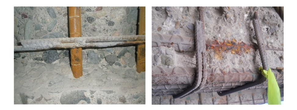
Includes repair of damaged reinforcing bars.
