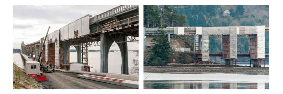
The north approaches of the bridge are receiving impressed current cathodic protection in a project that started in 2013. This project includes cathodic protection, Phase 1 seismic retrofit, expansion joint seal replacement, and larger bridge drains. "Stealth" rail and overlay were completed by change orders on the 2007-2012 project. Bid \$22.9 Million.
