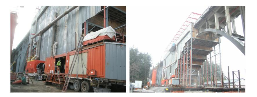
Includes work platforms and containment. A rigid frame work platform and containment system is shown with its heating and ventilating system.
