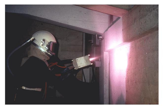
Includes abrasive blast surface preparation followed by arc-sprayed zinc coating of the concrete surfaces.
