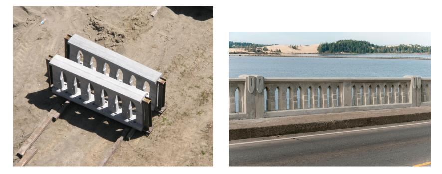
Since 2002 ODOT has been installing "stealth" railings on historic coastal bridges. The appearance of the original rail is replicated and strength is improved by embedding structural steel. A local precaster has built his business around this work.
