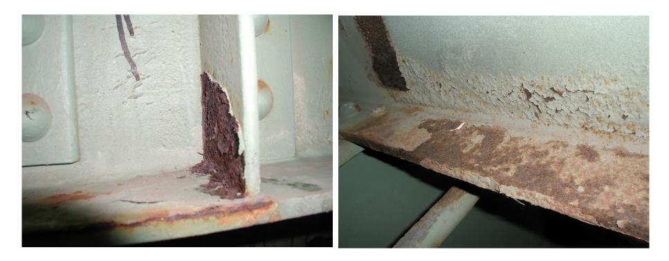
The bridge exists within 5 km of the Pacific Ocean. Marine salt damages the structural steel by providing an electrolyte and a catalyzing effect for corrosion.
