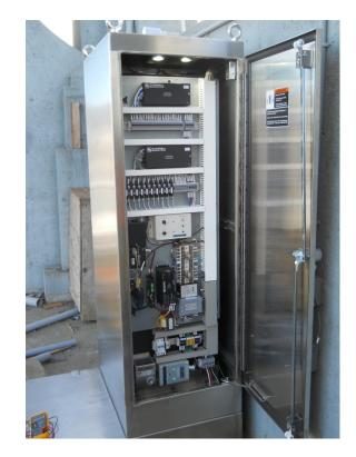
Includes installation of wiring and electrical equipment to power, control, and monitor the cathodic protection system.
