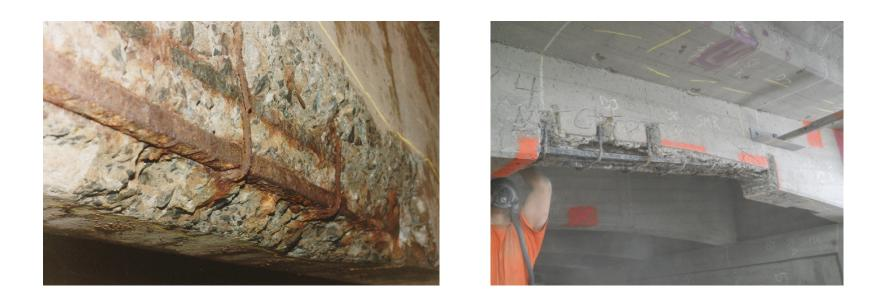
Includes removal of spalled and delaminated concrete
