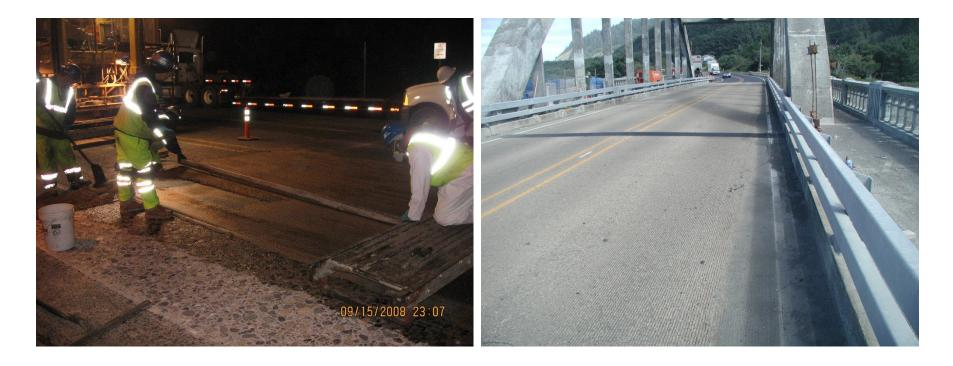
Roadway wearing surface is typically renewed with 19 millimeter (3/4 inch) thick premixed/screeded polyester polymer concrete over methacrylate primer, and expansion joint seals are typically replaced or retrofitted.
