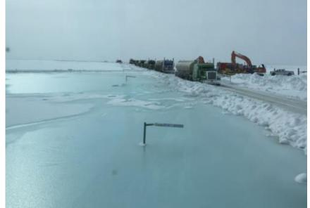
Dalton Hwy MP 396-405 - crews are working with Alyeska Pipeline Service Company to minimize overflow from the Sag River. The river is currently over the highway in eight locations, the largest spot is 12 inches deep and 200 feet long.
